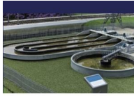
Treatment of Tannery Wastewater
